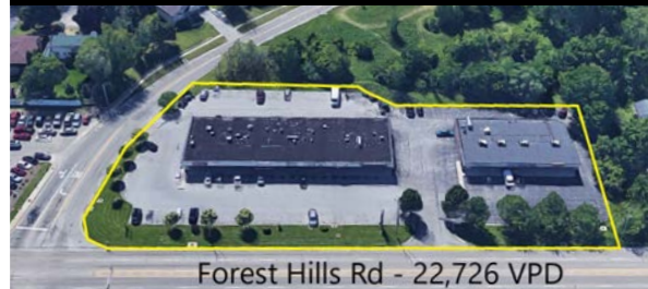
5811-61 Forest Hills Road, Rockford, IL
